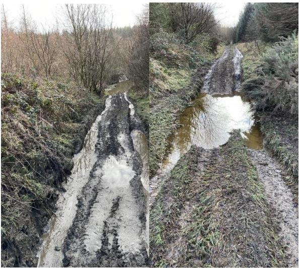
Photos 21 and 22 illustrate the poor access road condition from T5 south to T6, this is a wet area with crossing aquatic zones that are being damaged by quad use. Photo 22 also illustrates the location of T6 on the right-hand side within the Sitka spruce trees in plot 150.
