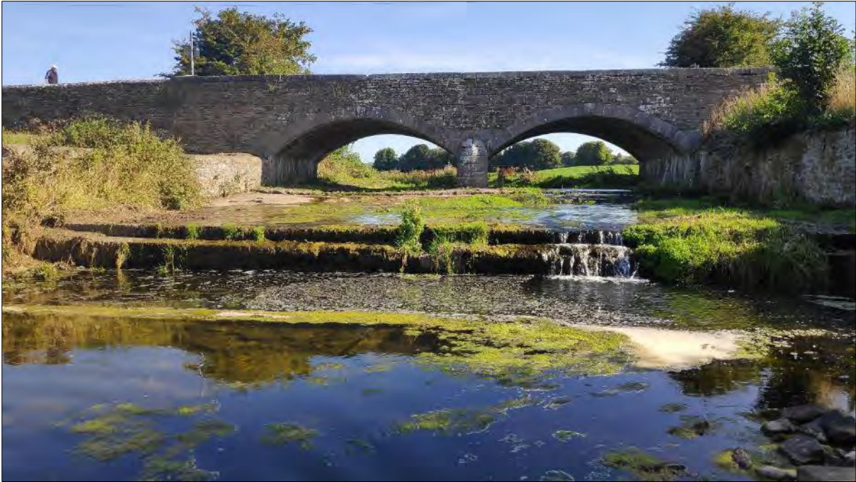
Plate 4.1 The historical weir at Clogh Bridge, an example of a significant barrier to fish passage at low flows
