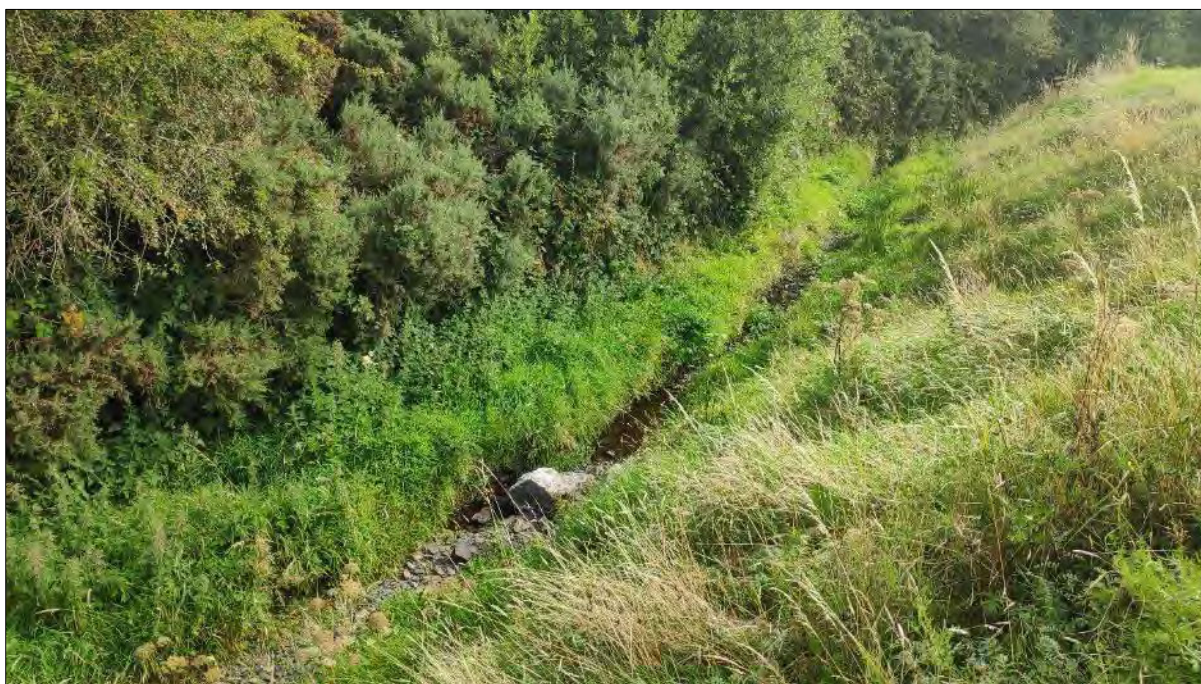
Plate 4.18 Representative image of site B2 on the upper reaches of the Owveg River, September 2022 (upstream of bridge)
