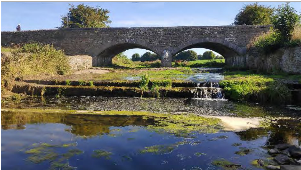
Plate 4.34 The historical weir at Clogh Bridge is a significant barrier to fish passage at low flows
