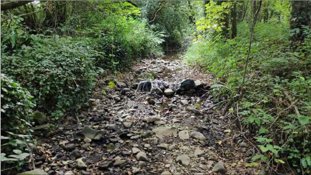
Plate 4.13 Representative image of site A12 on the Cremorgan Stream, September 2022 (upstream of bridge)
