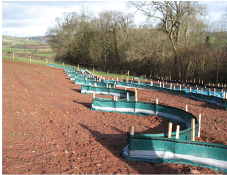
EXAMPLE OF INSTALLED SILT FENCING
