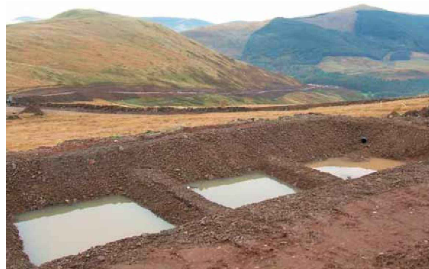
EXAMPLE OF CONSTRUCTED IN-LINE SILT TRAPS (FROM WIND FARM CONSTRUCTION GOOD PRACTICE GUIDE)
